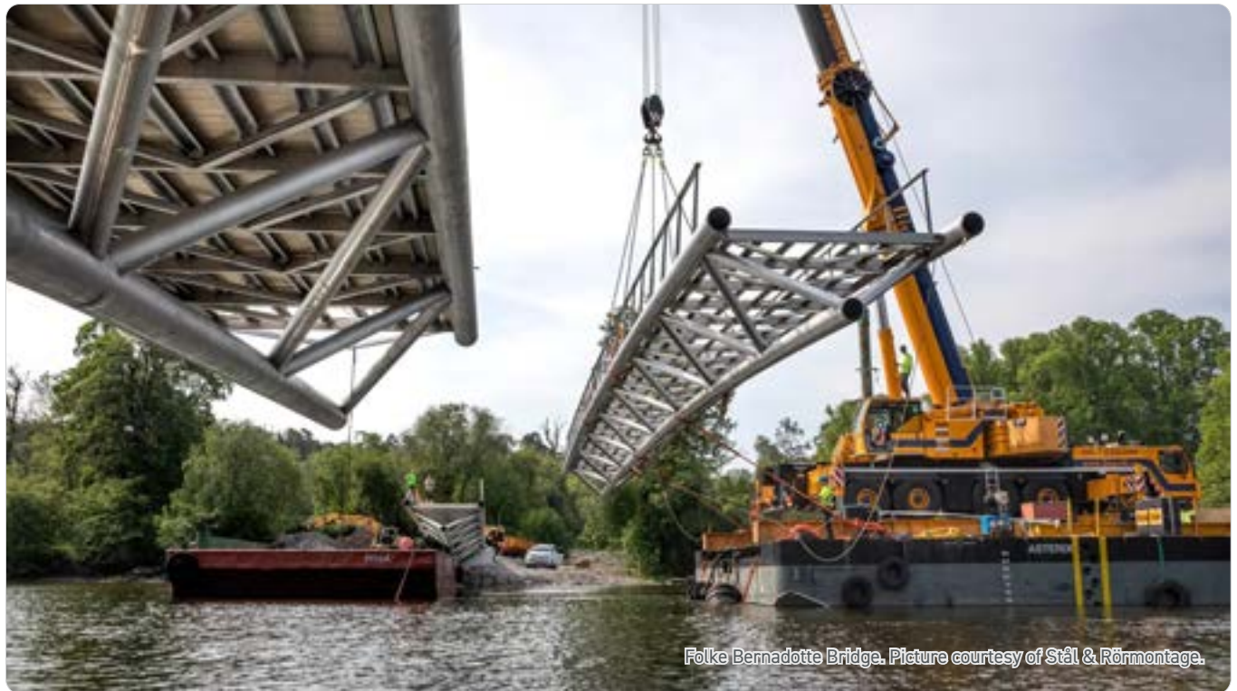
Folke Bernadotte Bridge. Picture courtesy of Stål & Rörmontage.
