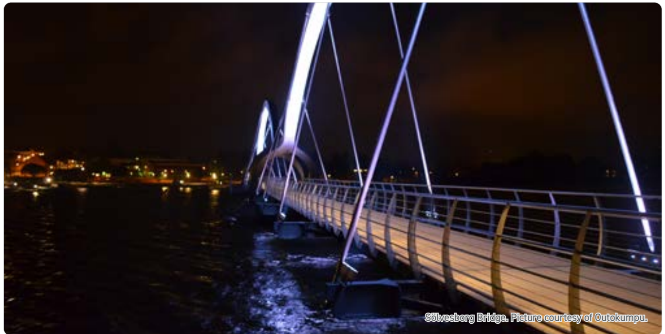
Sölvesborg Bridge. Picture courtesy of Outokumpu.
