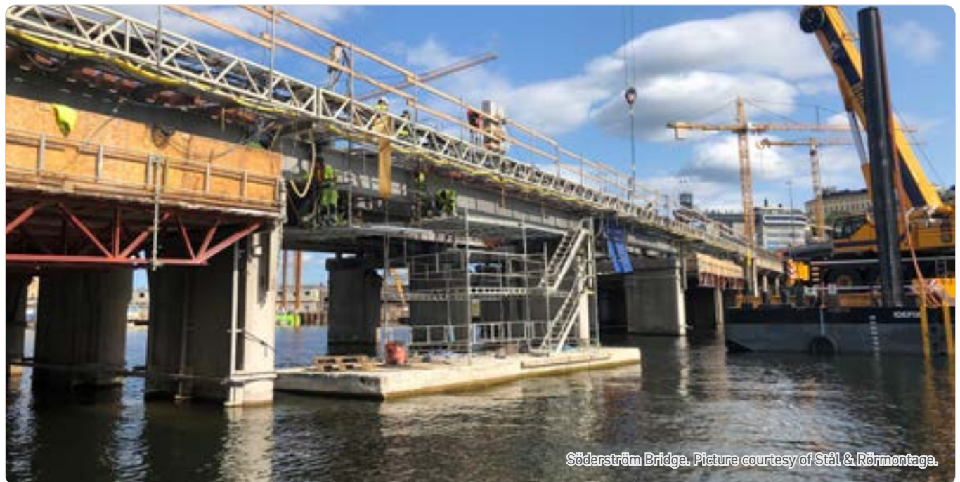
Söderström Bridge. Picture courtesy of Stål & Rörmontage.
